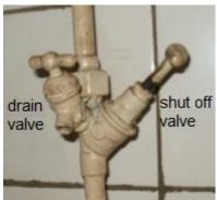
Step 2: Turn on the outside tap and the drain valve. As a result, all the water runs out of the pipe and cannot freeze to pieces. If necessary, blow the pipe empty if the water does not flow out by itself.
