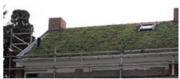
The block, which starts at Mgr. Poelsstraat 7, has been designated by the building association as a test object for the installation of "green" roofs. Sedum was chosen on top of the insulation of a thick sheet of PUR foam, instead of ordinary roof tiles. These are various types of very strong succulents and it insulates excellently. Good idea for the biodiversity in our neighborhood!
